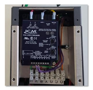
On the bottom left part of the ICM Fan Control, there is a label reading *N.C. Heat Pump* with an arrow pointing down to the 3-pin jumper. Remove the plastic jumper from the top two pins and push it into the bottom two pins or the center pin at the bottom. Doing this should result in the system transitioning into **Cooling Mode**, with the fan then proceeding to run at high speed.
