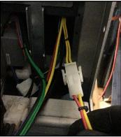
5. Firmly secure the ICM Delay to the unit with the double-sided Foam Tape provided.
