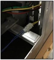
3. Disconnect the two High-Pressure Sensor Wires from the corresponding Yellow Wires by squeezing the release tabs, then plug the Male side of the Anti-Ice Freeze Stat (Yellow & Black Wires) into the Female plug off the High-Pressure Sensor.
